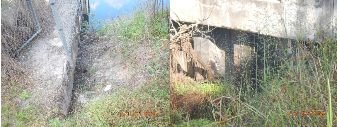
Erosion upstream of Structure sheetpile
