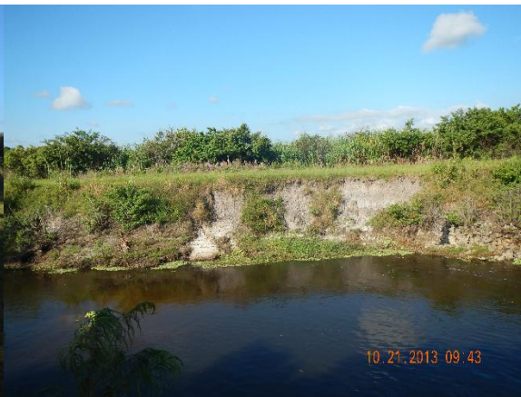
Downstream Bank Erosion
