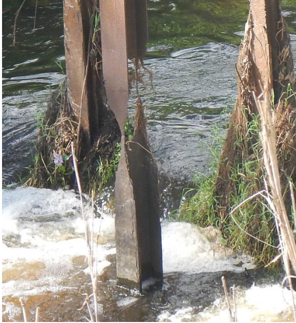
Structural components rusted through Discharge
