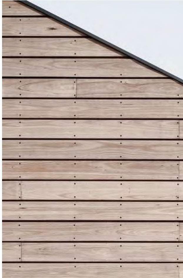
Open jointed horizontal timber cladding, bandsawn finish
